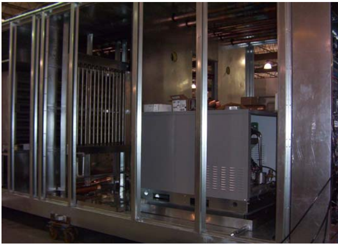
900 LB/HR natural gas-fired self-contained humidifier with modulating controls.
