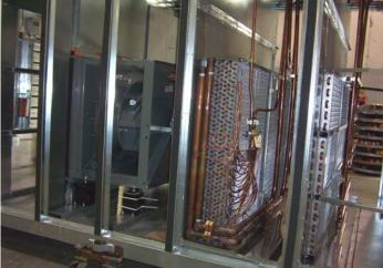
The cooling sections consist of HCFC- free R-410A refrigerant with three (3) scroll compressors piped to 3 independent intertwined DX coils with 3 hot gas reheat coils.
