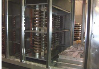
Some of the features include outside air flow monitoring stations, airfoil SWSI plenum supply and return air blowers, premium efficiency motors and VFDS, tubular type gas burners with SS heat exchangers, and supply and return smoker dampers.
